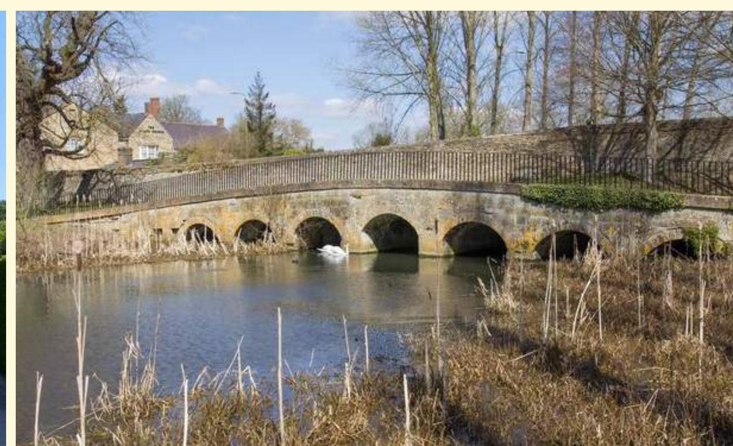
Seven Arches Bridge, Grade II Listed
